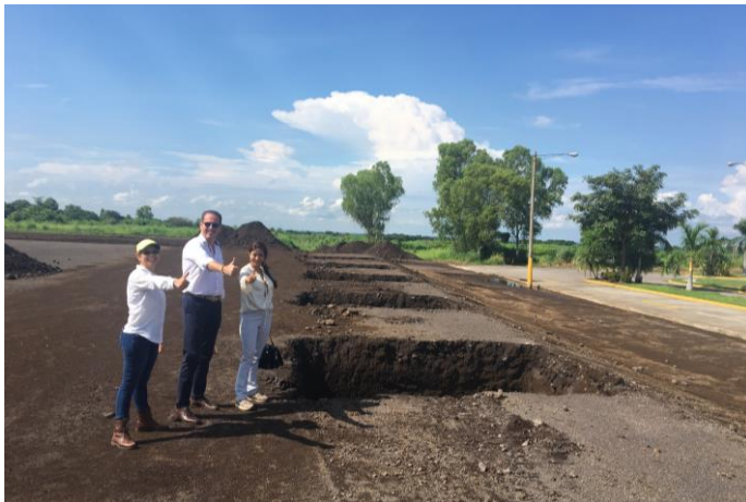
Construction work starts
